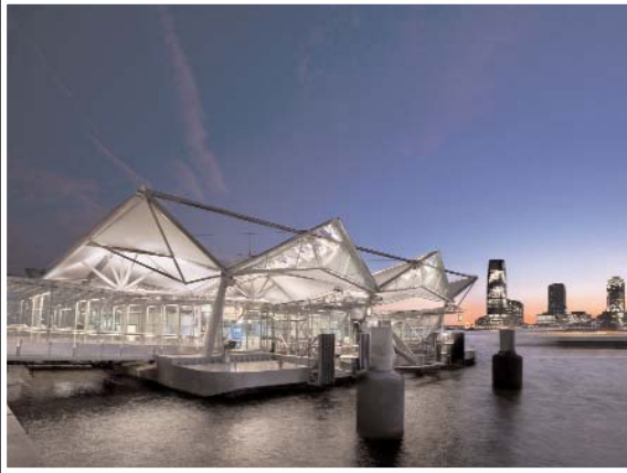
The Port Authority Ferry Terminal at World Financial Center The Port Authority of NY & NJ Design Division
