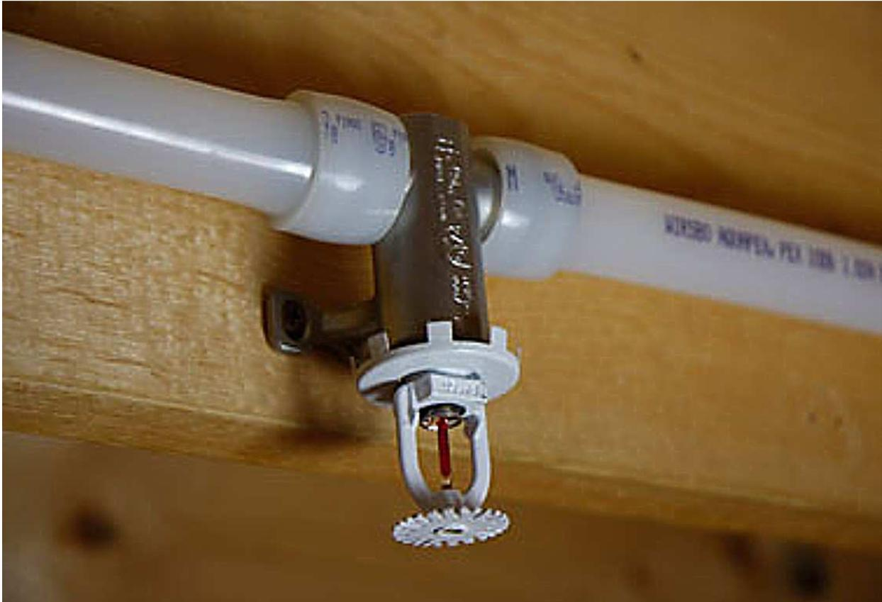
*Image of a residential type fire sprinkler head and pipe (NFPA 13R system)*
