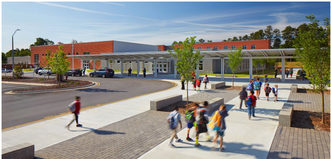
A critical design element in school safety is addressing the building entry. By funneling visitors to a single point of entry and creating a vestibule within that entry where they can be greeted and identified, the school can better control access and safety.
